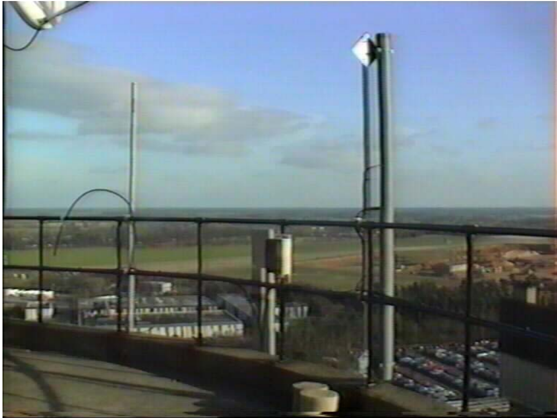
Fig 12 GB3MHS Antenna Installation
